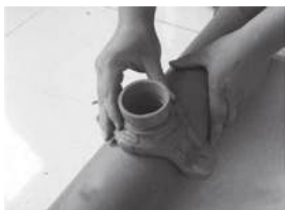
4. Install the Mechanical Tee in the hole.
