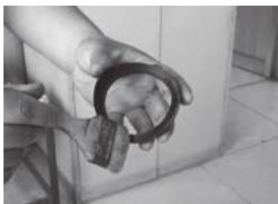
2. Spread lubricant on gasket ring.
