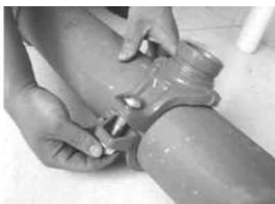
5. Install the bottom piece on the upper one of Mechanical Tee.
